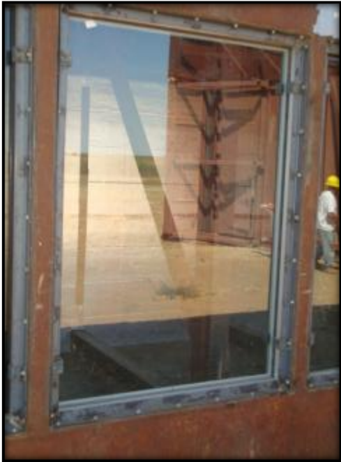
Figure C.17: L6 Pre-Blast Condition
