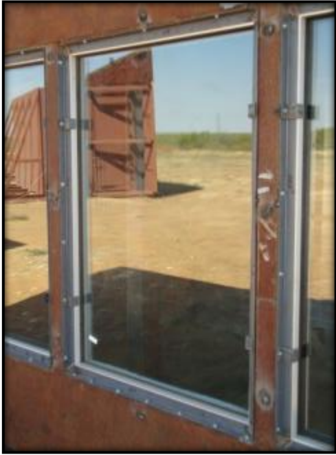
Figure C.5: L3 Pre-Blast Condition
