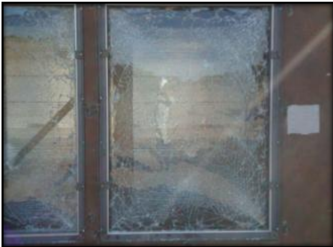
Figure C.11: L4 External Post-Blast Condition
