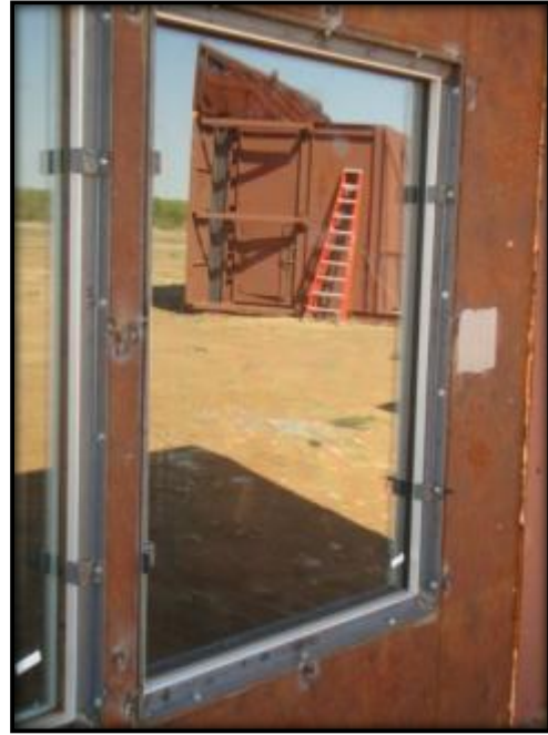
Figure C.6: L4 Pre-Blast Condition
