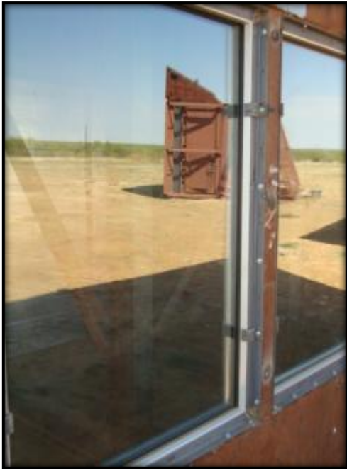
Figure C.3: L1 Pre-Blast Condition
