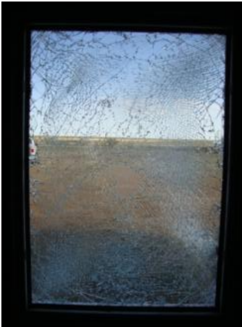
Figure C.15: L4 Internal Post-Blast Condition
