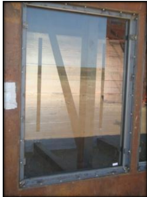
Figure C.16: L5 Pre-Blast Condition
