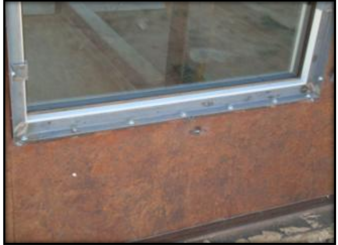
Figure C.2: L1 Bolt Connection Pre-Blast Condition
