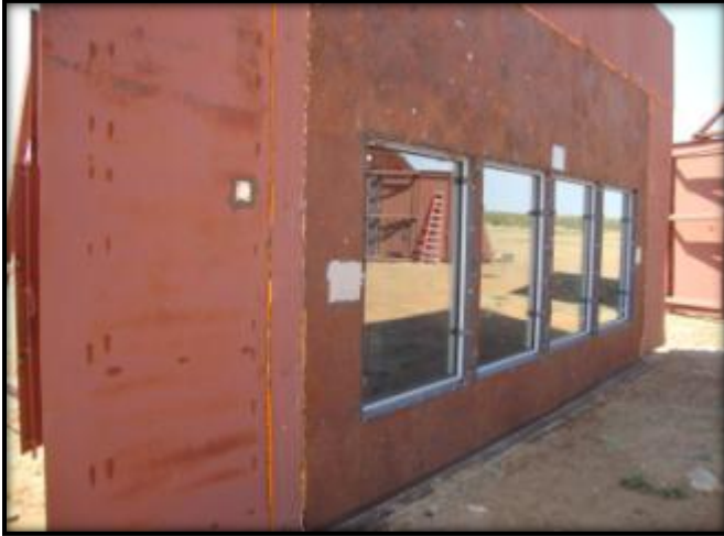
Figure C.1: Chamber 1 Pre-Blast Condition
