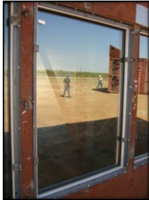
Figure C.4: L2 Pre-Blast Condition
