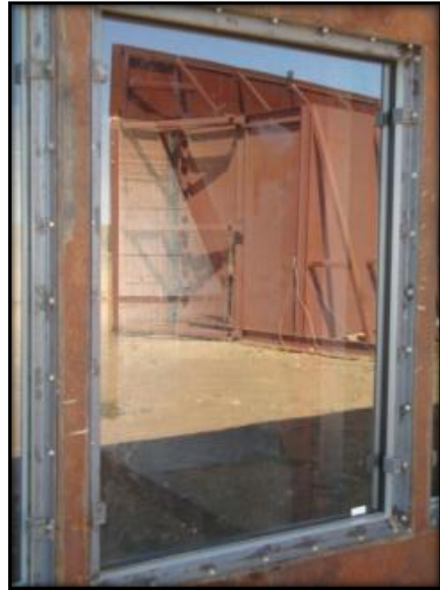
Figure C.18: L7 Pre-Blast Condition
