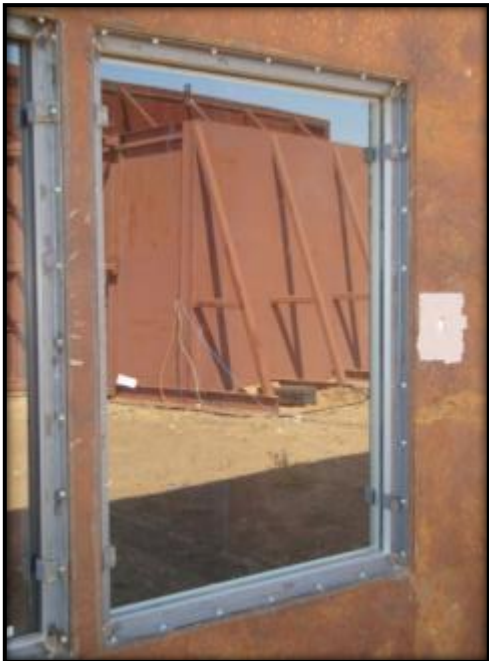
Figure C.19: L8 Pre-Blast Condition
