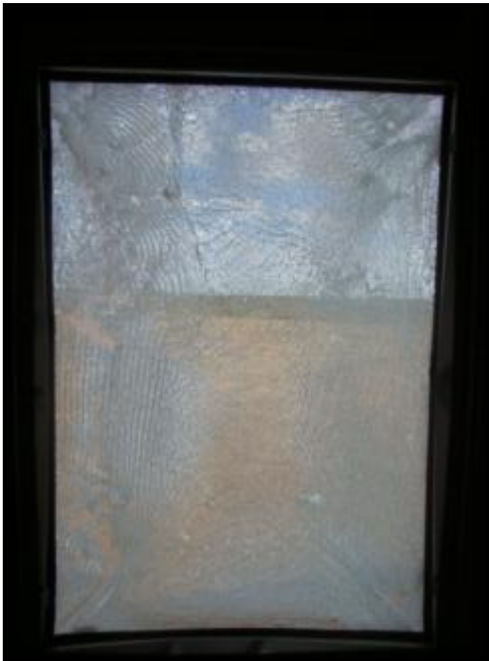
Figure C.35: L7 Internal Post-Blast Condition
