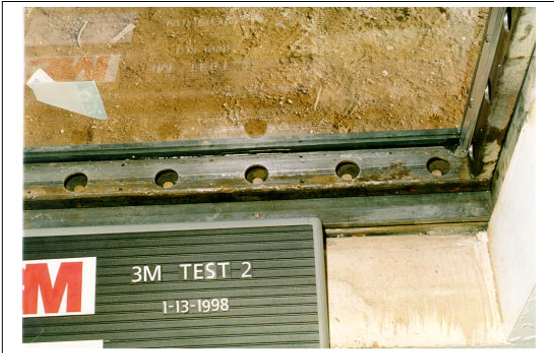
Figure A.76. Test 2. Pretest, interior view of window 4. Close-up view of the batten system (3M T2 PRE 01.tif).
