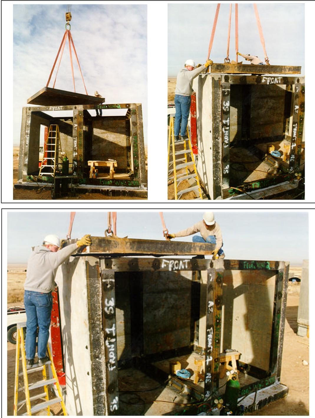
Figure A.3. Placement of the South Bay Structure roof panel (3M PREP 20.tif, 3M PREP 19.tif, 3M PREP 17.tif).
