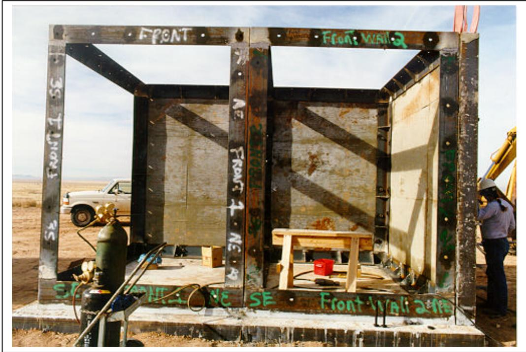
Figure A.1. The steel frame of the modular reaction structure (viewed from the east face) (3M PREP 15.tif).
