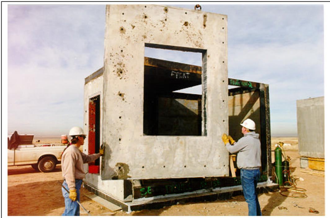
Figure A.5. Placement of the South Bay Structure front panel into the modular structure steel frame (3M PREP 03.tif, 3M PREP 04.tif).
