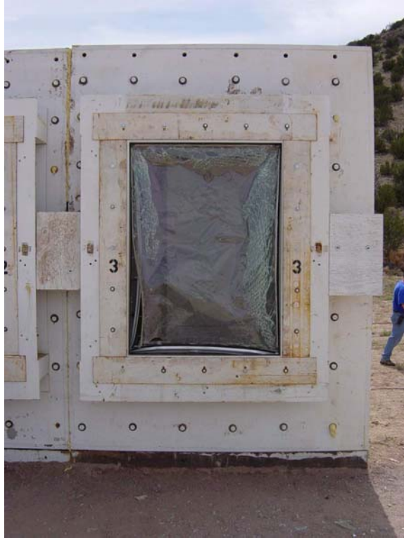
Figure 3-9 Exterior post-test view of window 3. (DSC04059.jpg)
