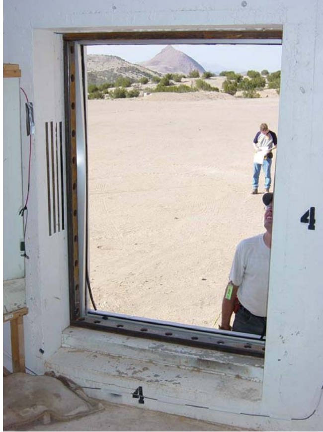
Figure 3-65 Interior post-test view of window 4. (DSC04567.jpg)
