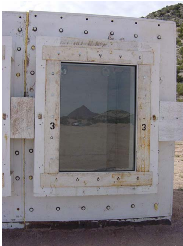
Figure 3-34 Exterior pre-test view of window 3. (DSC04249.jpg)
