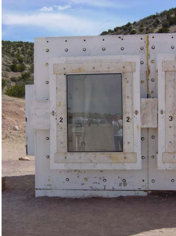
Figure 3-57 Exterior pre-test view of window 2. (DSC04456.jpg)
