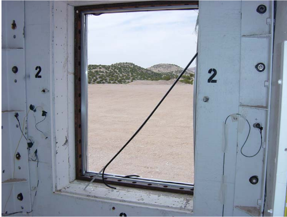
Figure 3-20 Interior post-test view of window 2. (DSC04189.jpg)
