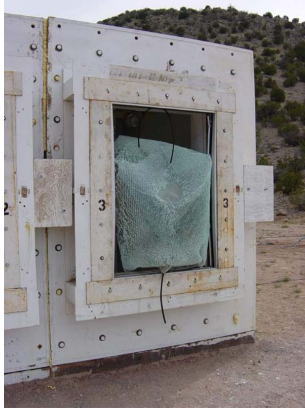
Figure 3-22 Exterior post-test view of window 3. (DSC04162.jpg)
