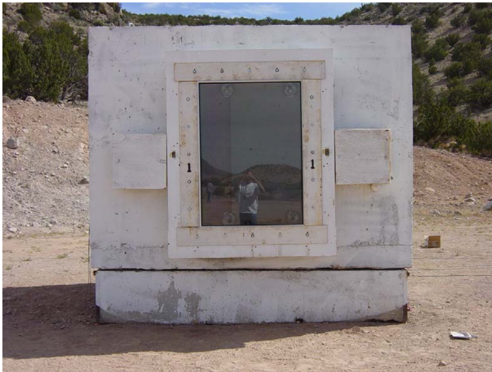
Figure 3-54 Exterior pre-test view of window 1. (DSC04446.jpg)
