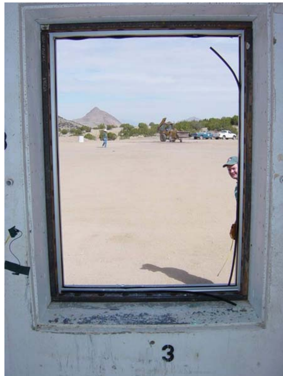
Figure 3-36 Interior post-test view of window 3. (DSC04318.jpg)
