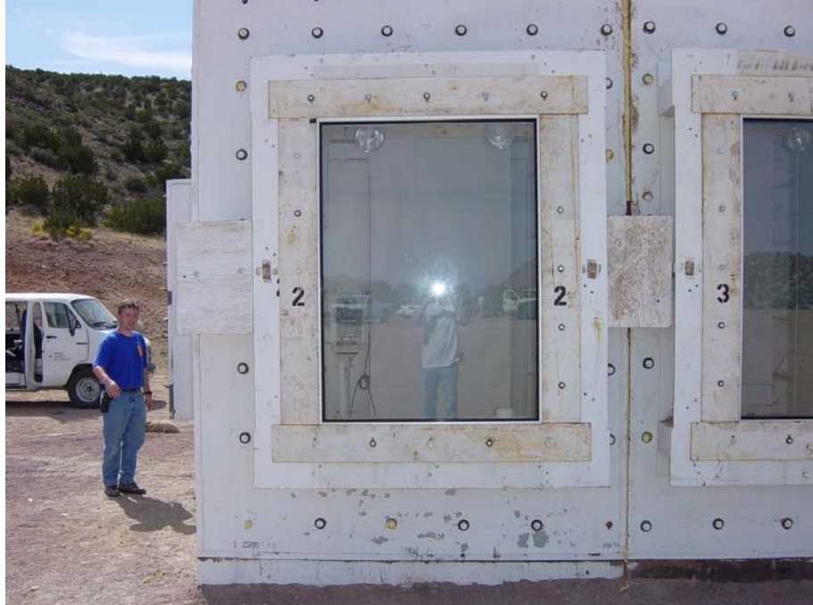
Figure 3-5 Exterior pre-test view of window 2. (DSC04001.jpg)
