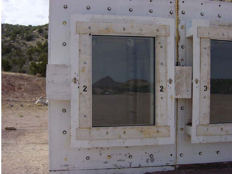
Figure 3-31 Exterior pre-test view of window 2. (DSC04248.jpg)
