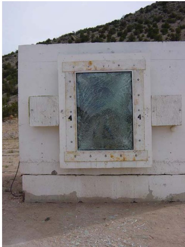
Figure 3-25 Exterior post-test view of window 4. (DSC04214.jpg)
