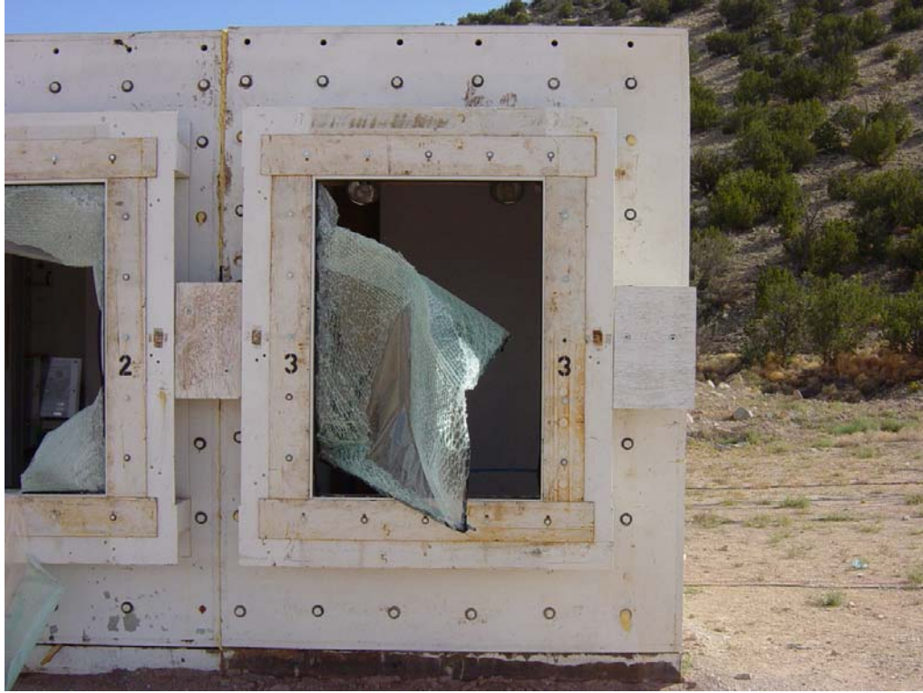
Figure 3-61 Exterior post-test view of window 3. (DSC04493.jpg)
