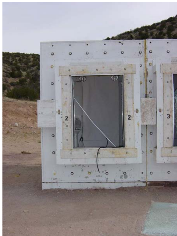
Figure 3-19 Exterior post-test view of window 2. (DSC04178.jpg)
