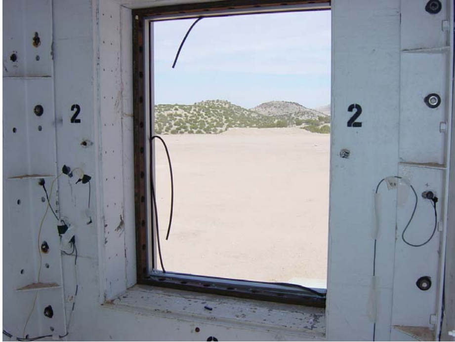
Figure 3-33 Interior post-test view of window 2. (DSC04304.jpg)
