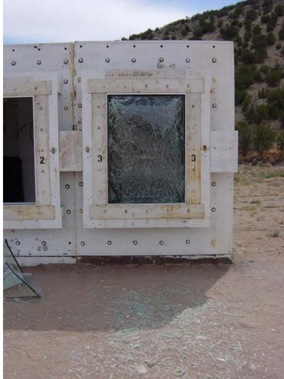
Figure 3-48 Exterior post-test view of window 3. (DSC04367.jpg)
