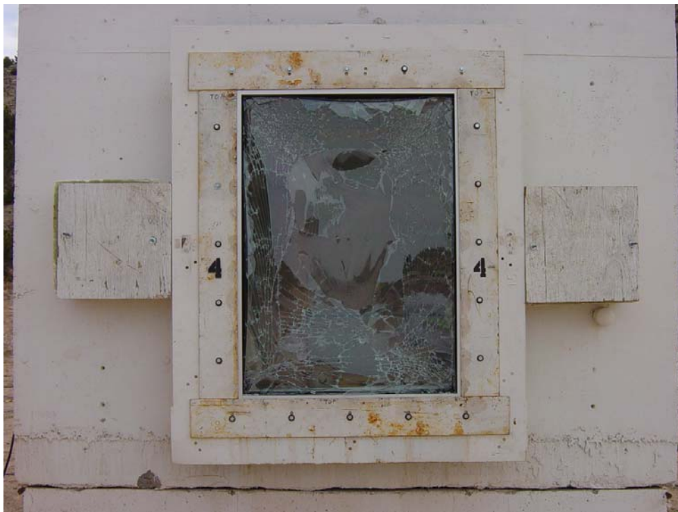
Figure 3-12 Exterior post-test view of window 4. (DSC04084.jpg)
