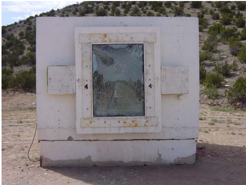
Figure 3-38 Exterior post-test view of window 4. (DSC04330.jpg)
