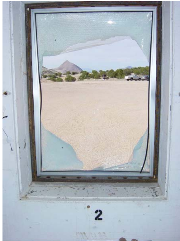
Figure 3-59 Interior post-test view of window 2. (DSC04533.jpg)
