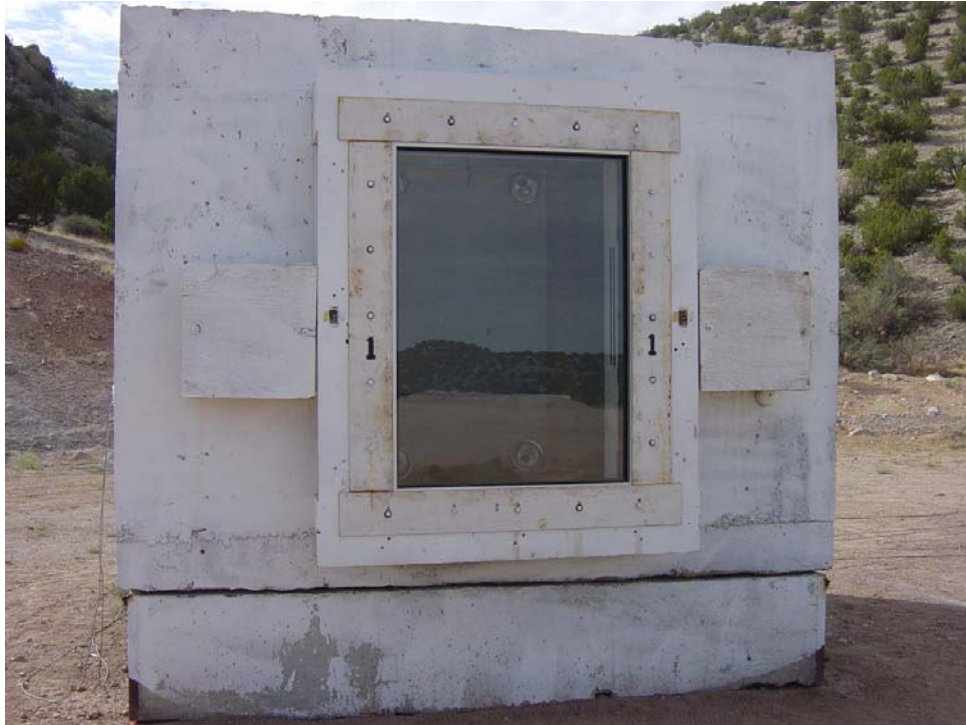
Figure 3-28 Exterior pre-test view of window 1. (DSC04237.jpg)
