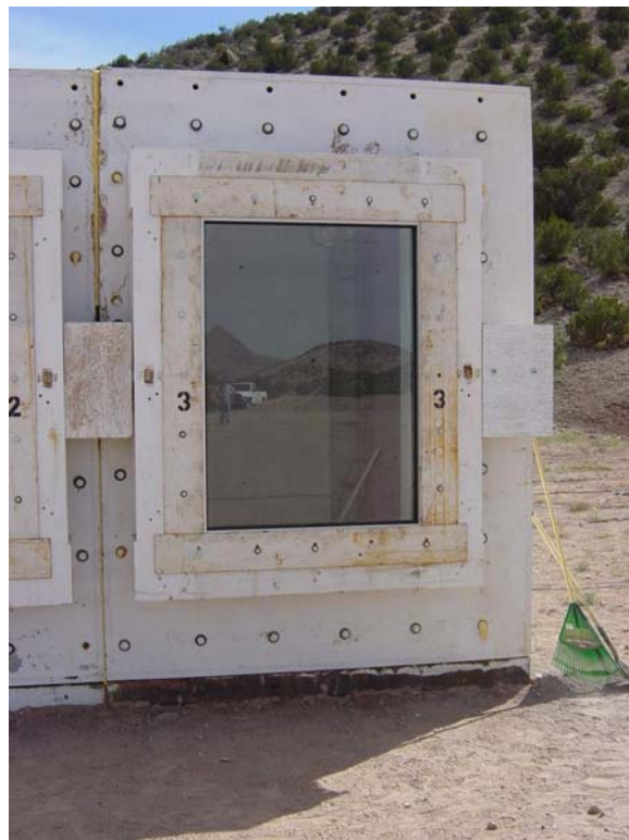
Figure 3-60 Exterior pre-test view of window 3. (DSC04460.jpg)
