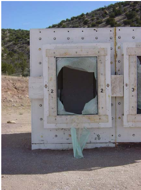
Figure 3-58 Exterior post-test view of window 2. (DSC04497.jpg)
