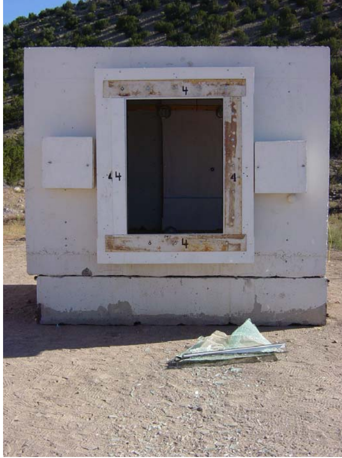
Figure 3.13. Exterior post-test view of Window 4.
