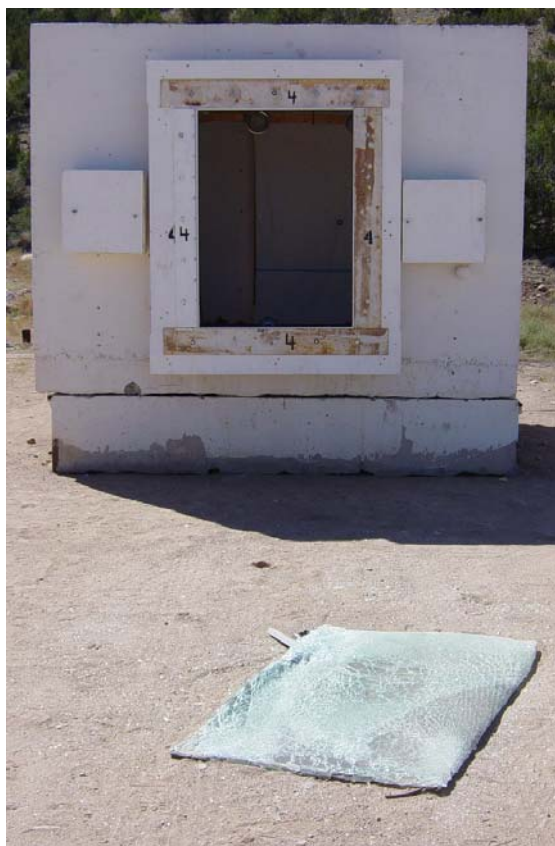
Figure 3.26. Exterior post-test view of Window 4.
