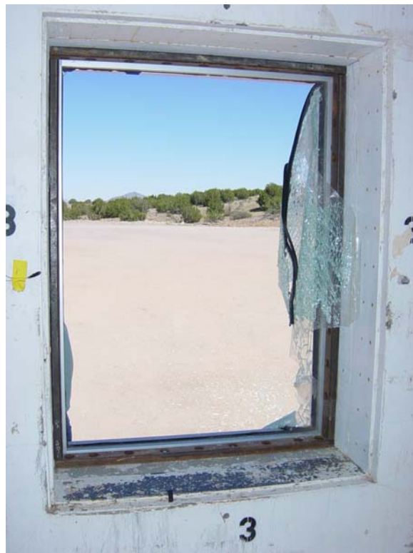
Figure 3.22. Interior post-test view of Window 3.
