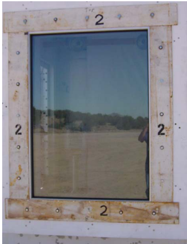
Figure 3.5. Exterior pre-test view of Window 2.
