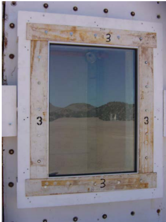
Figure 3.21. Exterior pre-test view of Window 3.
