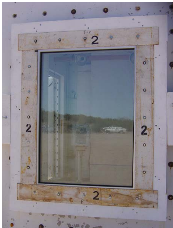
Figure 3.18. Exterior pre-test view of Window 2.
