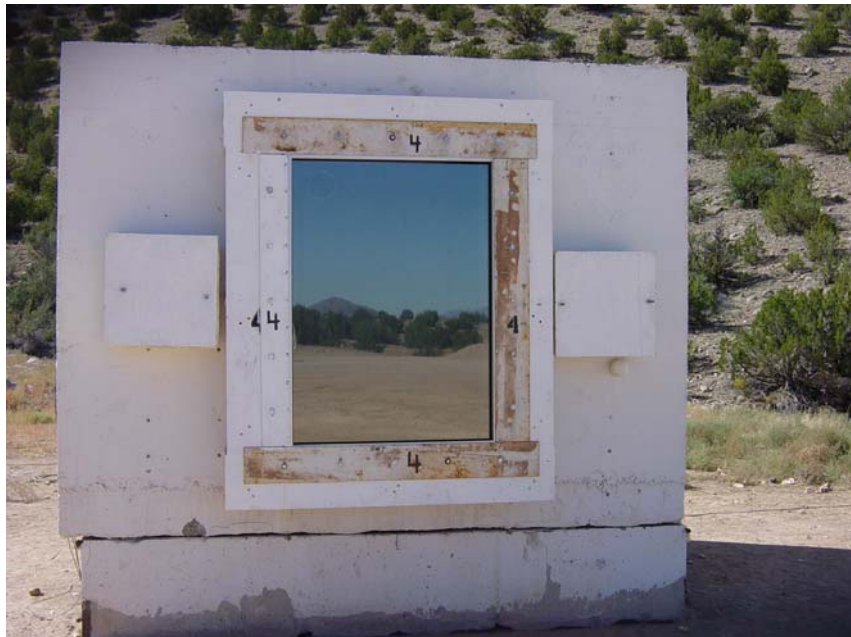
Figure 3.24. Exterior pre-test view of Window 4.
