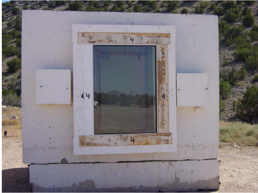
Figure 3.11. Exterior pre-test view of Window 4.
