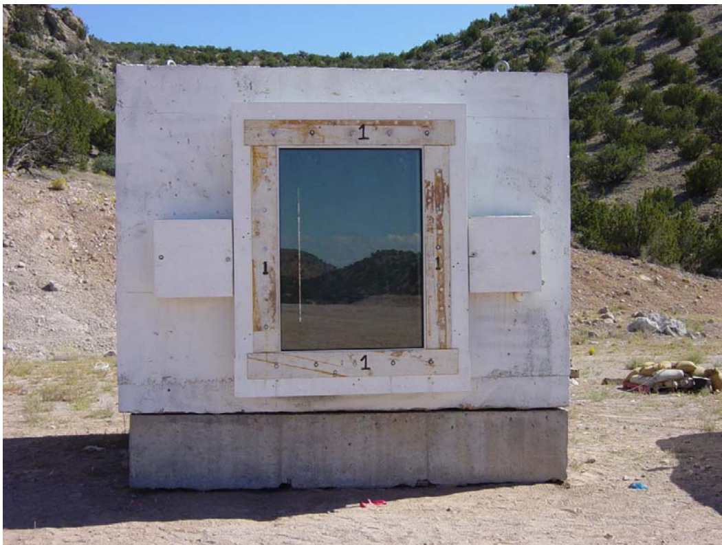
Figure 3.2. Exterior pre-test view of Window 1.
