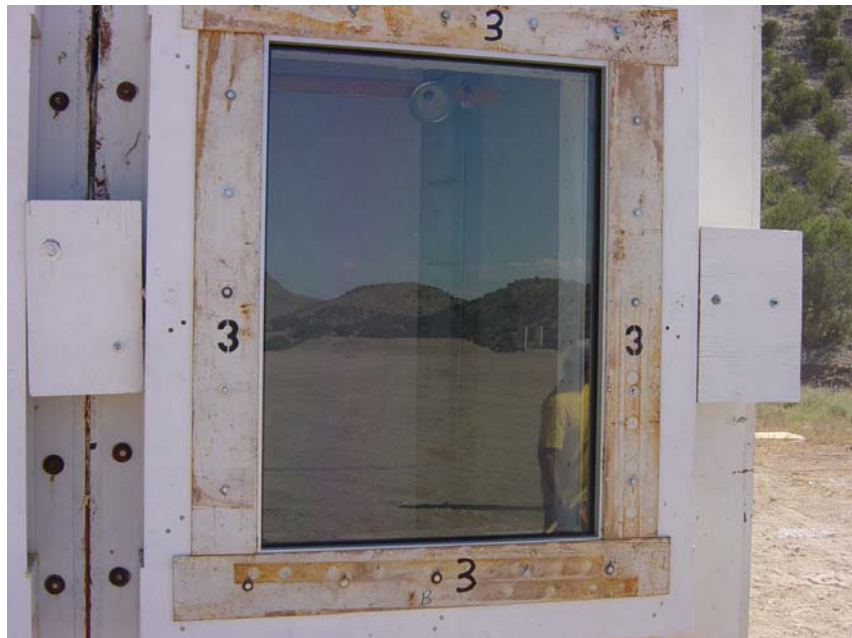
Figure 3.8. Exterior pre-test view of Window 3.
