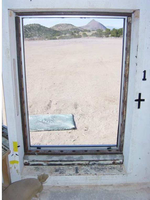
Figure 3.3. Exterior post-test view Window 1.
