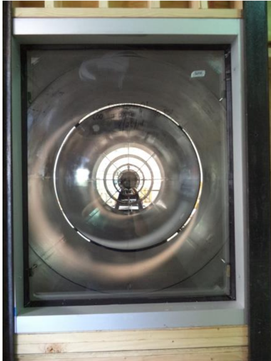
Photo No. 25 Pre-test Specimen #9, Interior
