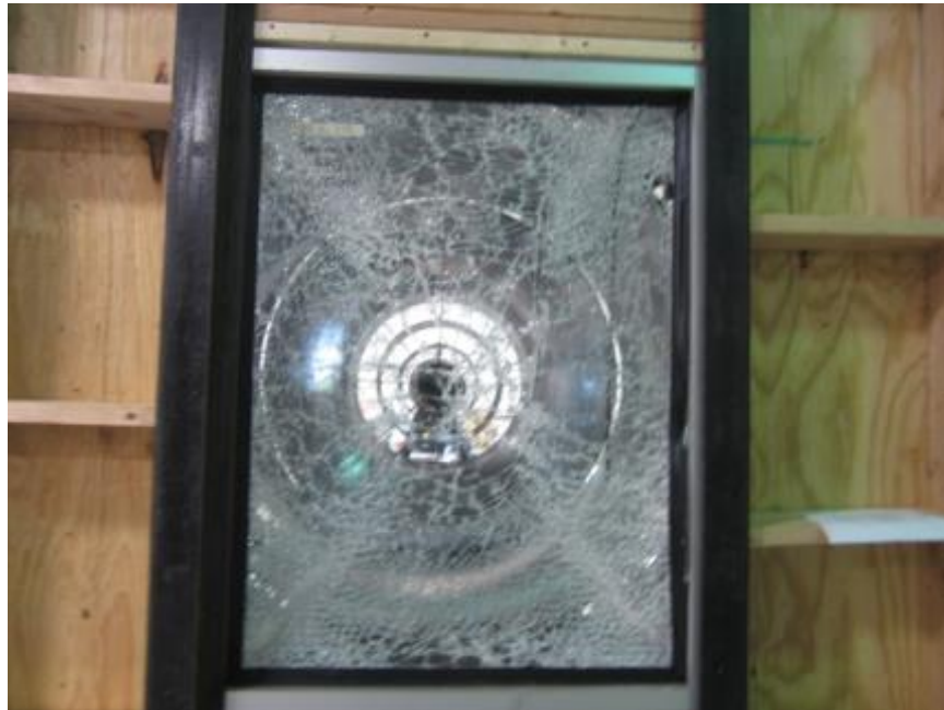
Photo No. 25 Post-test Specimen #9, Interior
