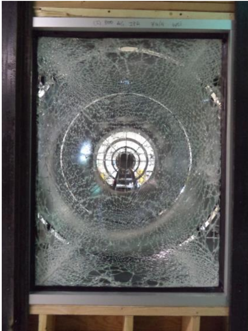
Photo No. 34 Post-test Specimen #13, Interior
